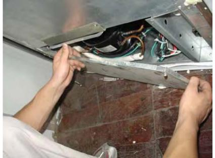
3. Remove the screws from the control board cover.
